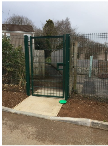
A new Year six entrance at the back of the school.
